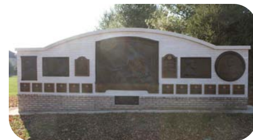
(The Masonic Memorial Wall in completion)
